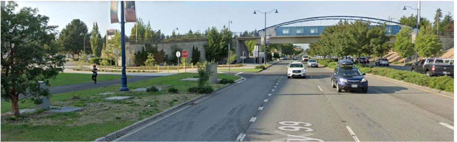
Photo: Google Street View
