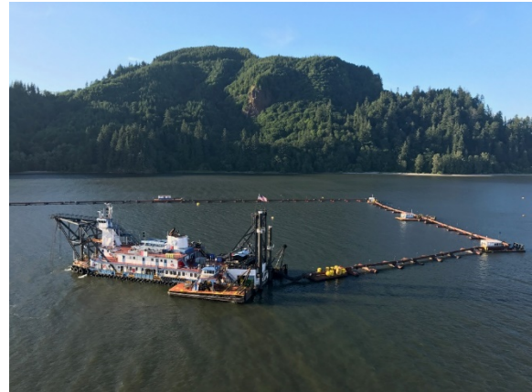
Dredging near Longview. Photo: Port of Longview
